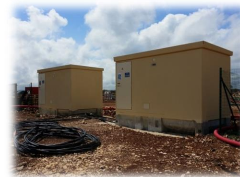
Pose de postes HTA
